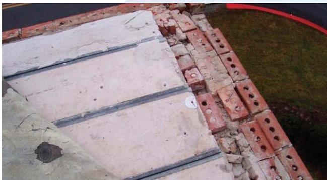
Not surprisingly, our investigation revealed inadequate perimeter construction with wood blocking fastened directly to the top course of brick. This configuration prevented adequate resistance to wind forces resulting in the failure observed.
