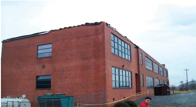
This roof in western North Carolina was blown off due to high winds not associated with a storm. Bricks, wood blocking, sheet metal and membrane were blown over 100 feet across an adjacent courtyard.
