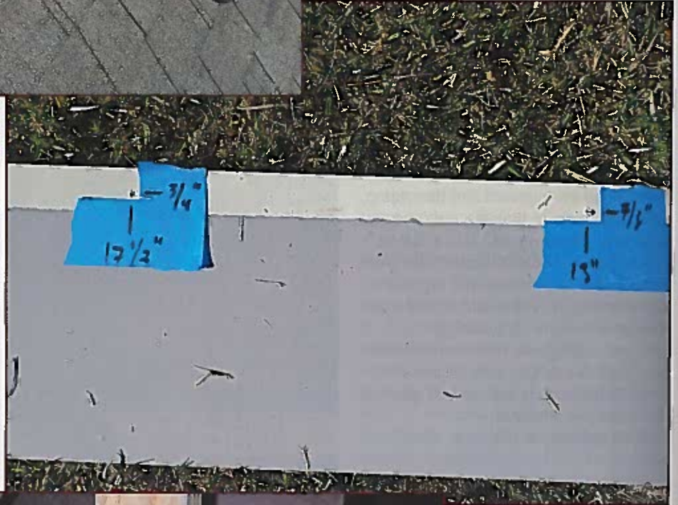
Figure 5 – Cementitious siding horizontal spacing.
