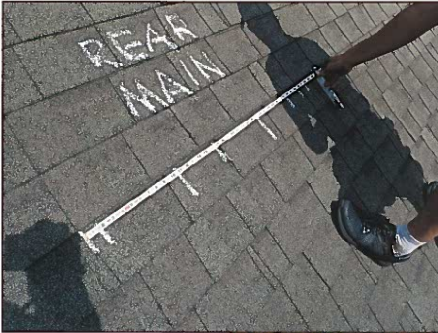
Figure 4 – Roof shingle horizontal spacing.
