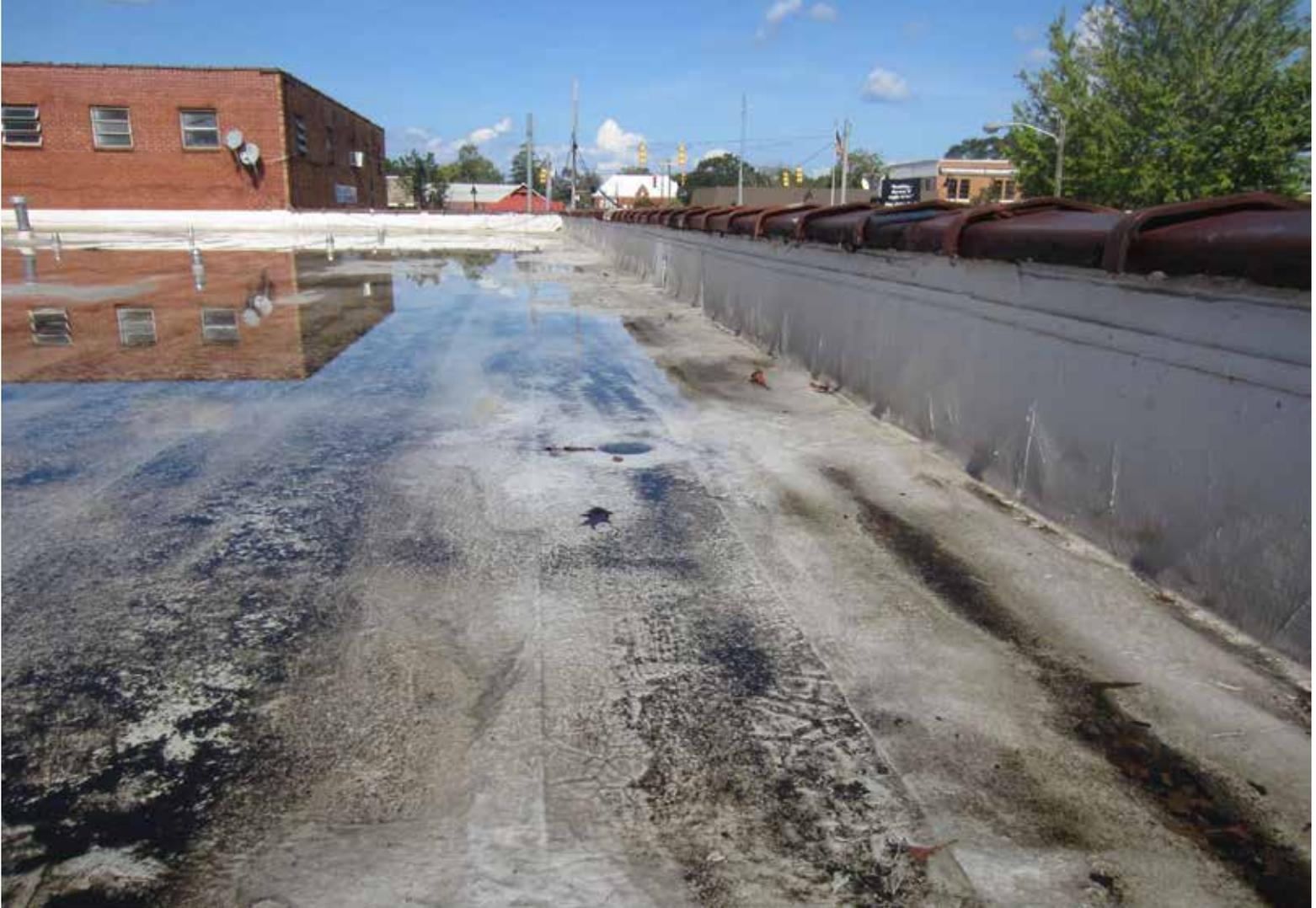
Standing water is a primary source of roof cover discoloration and deterioration that may result in framing member damage and contribute to premature failure of the structural system on low-slope roofs.
